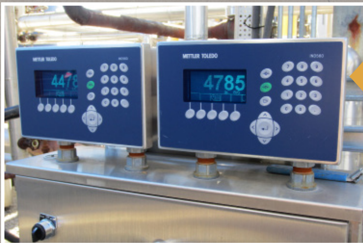
Controllers are IND560 controllers (one per each scale, 120-volt power). Include optional discrete I/O output to turn pump off at end of injection.
