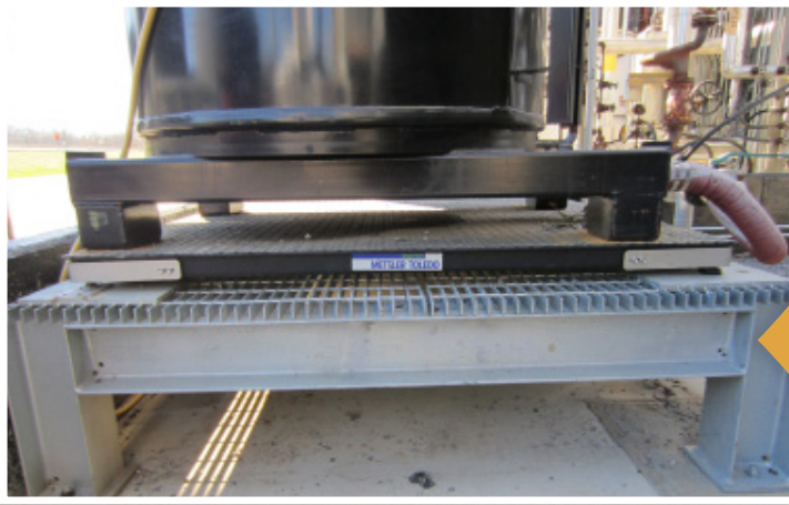
Scales are typically Mettler Toledo VLC floor scales (5,000 lb capacity).
