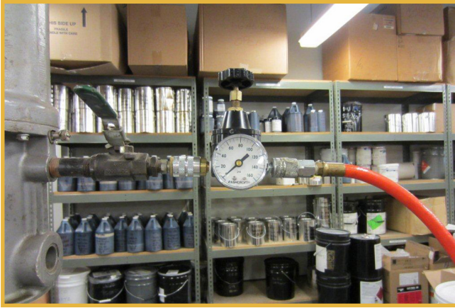
On the inlet side of the pump, an air regulator controls inlet air pressure.
