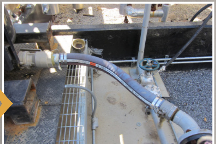
Utilize short truck hose between totes and pump so that scale is isolated from piping and equipment weight/forces.
