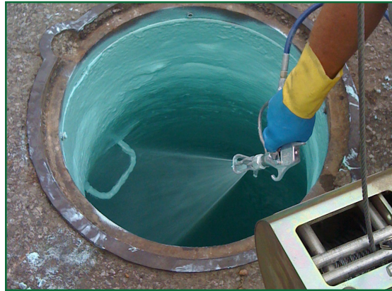
Novocoat SG2500 Lining high build epoxy application.
